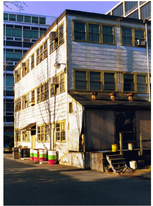
View of shed extending of the south end of A Wing."
