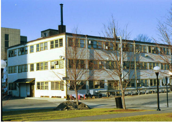
Building 20, view of the east side of C Wing, 1997.
