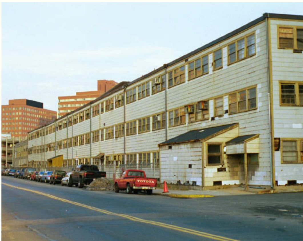
Building 20, Vassar Street facade, 1997.
